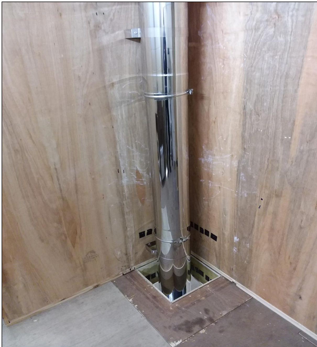
Figure 4 – Twin wall system chimney through Zone B
