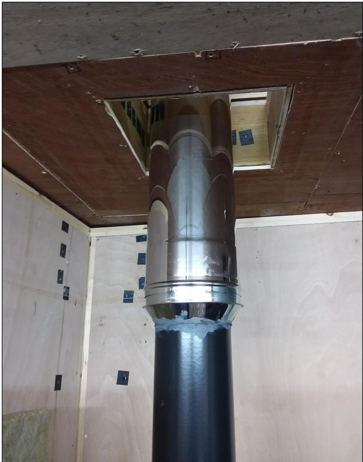
Figure 3 – Connection to twin wall chimney
