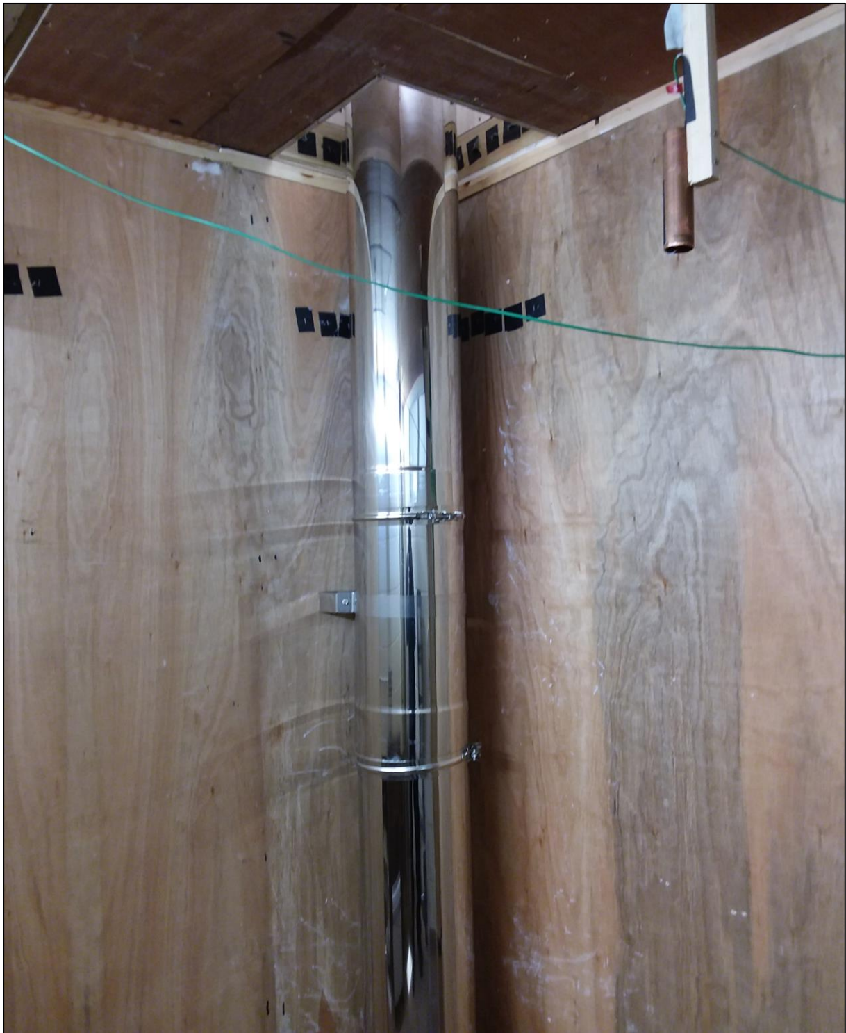
Figure 5 – Twin wall system chimney through Zone B ceiling
